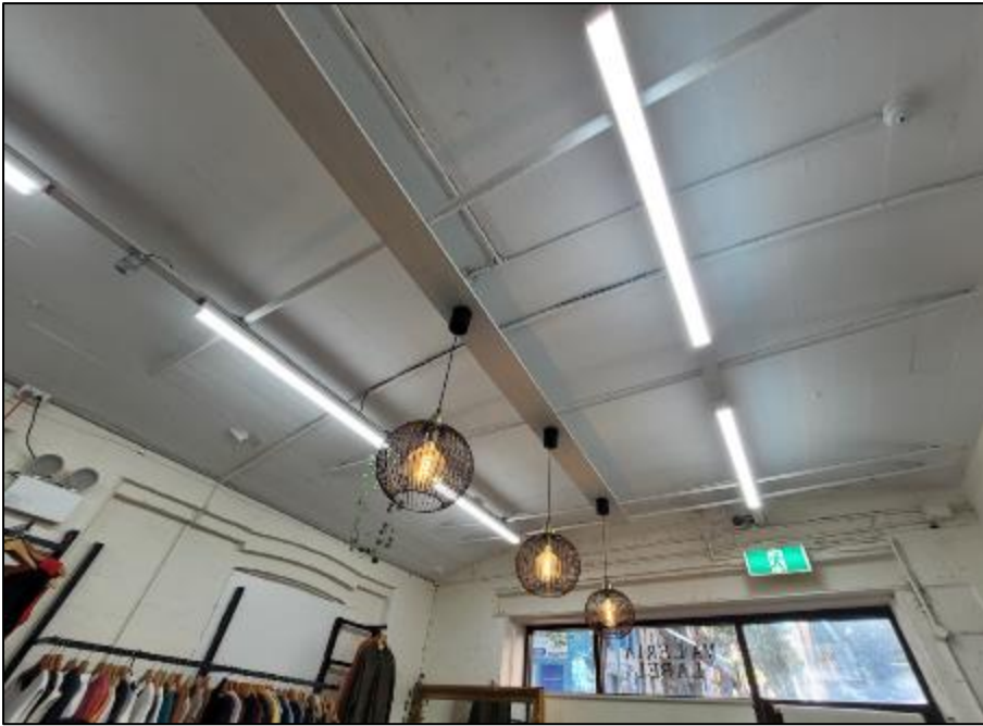
Figure 8: Existing arched vaults in the ground floor retail tenancy
