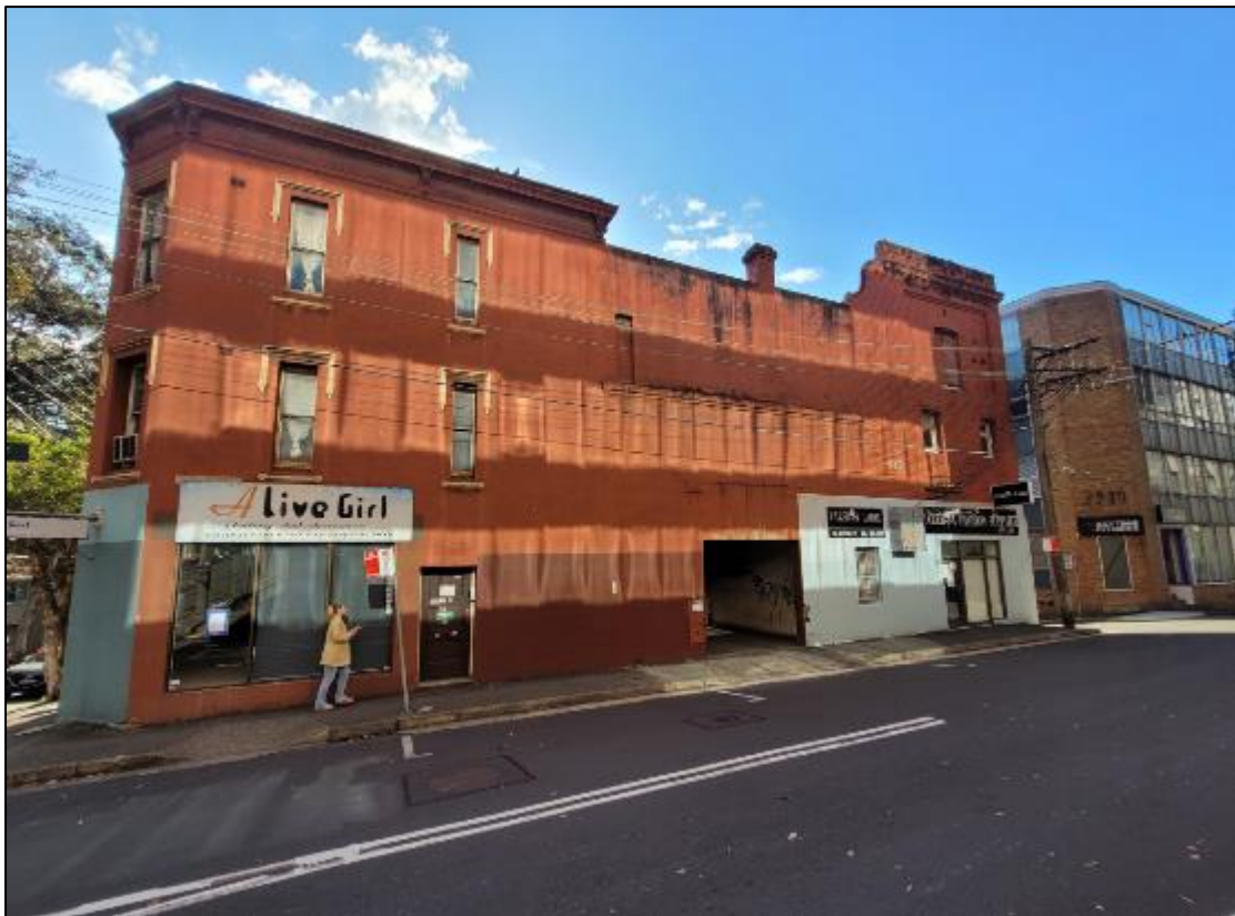
Figure 3: Site viewed from Waterloo Street
